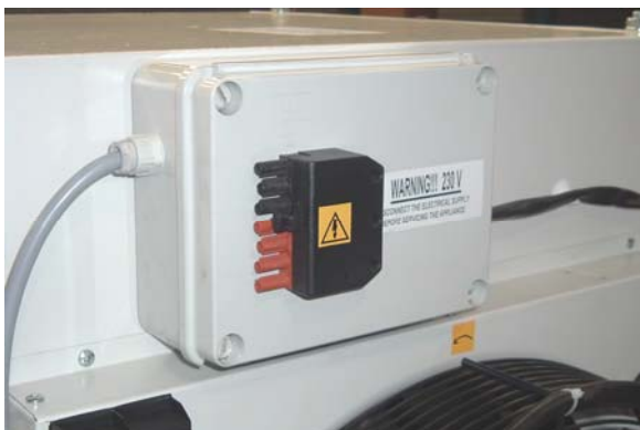
fig.1 – Heater control cover & fixed socket
