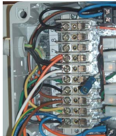
fig.3 – Terminal strip. *OFSU 100 has an additional plastic terminal (not shown)
