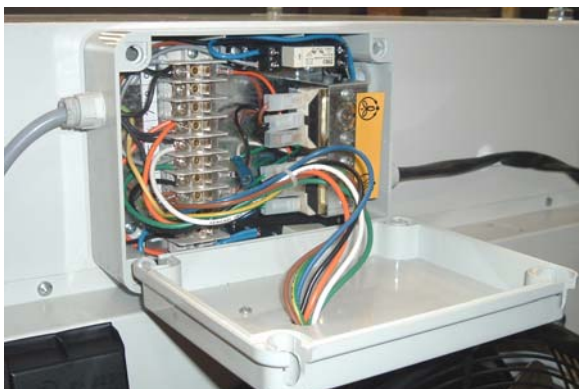
fig.2 – Opened control panel.
