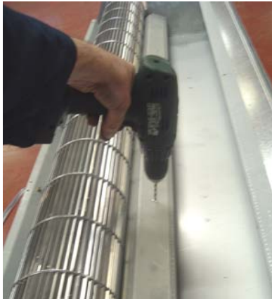
fig.6— Removal of deflector plate
