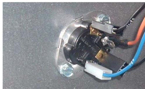
fig.3 - Typical Fan Control in situ
