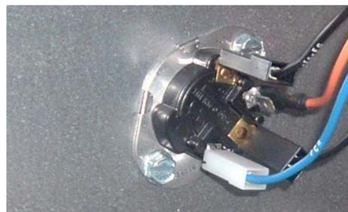
fig.3 - Typical Fan Control in situ
