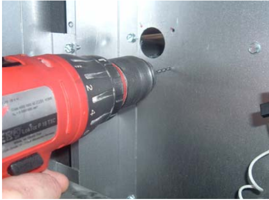
fig.15 - drilling 4 holes
