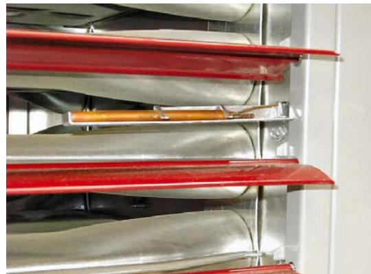
fig.26 - capillary bulb positioning
