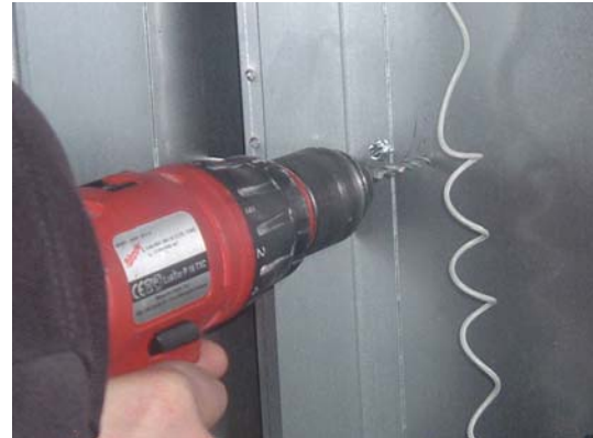
fig.12. - drilling a pilot hole.
