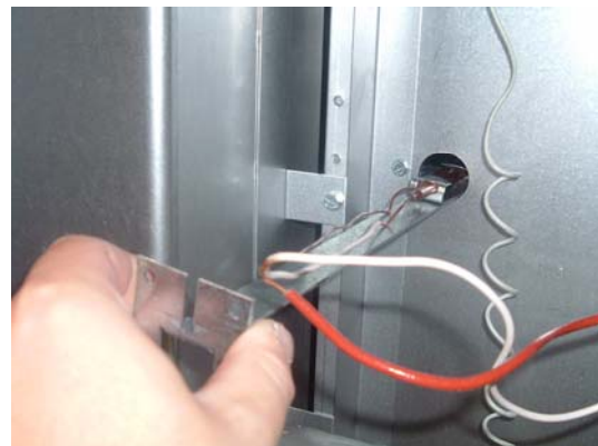
fig.13 - replacement limit 'bulb' orientation
