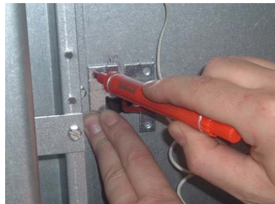
fig.14 - marking using template
