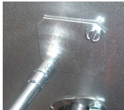
fig.19 - fixing blanking plate over original LC1 hole
