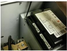
6) Connect the Pactrol, valve plug and earth
