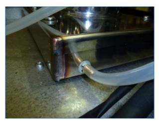
Feed the tubing through the gland on top of the burner housing, cut to length, then fit to the air pressure switch positive spigot as shown.
