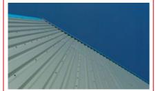
CA Groups SolarWall<sup>®</sup> is an astonishingly simple, effective solution to the demand for  $CO_2$  reduction - and the energy cost savings that accompany it. A steel or aluminium cladding for industrial and commercial buildings that captures warmth from the sun and uses solar heated air to heat the building.
