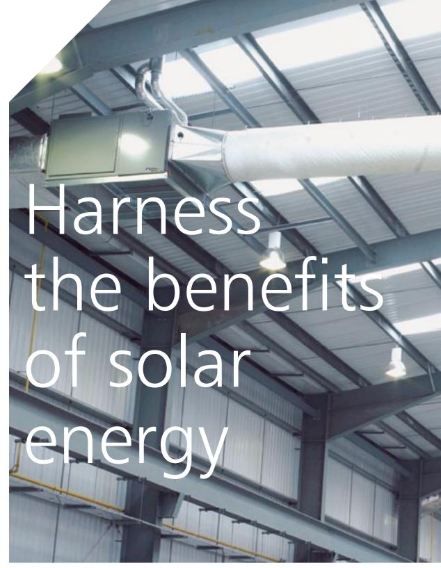
Systems can be matched to applications as diverse as full heating or tempered make-up air, in each case optimising the use of solar heated air produced by the SolarWall®.
