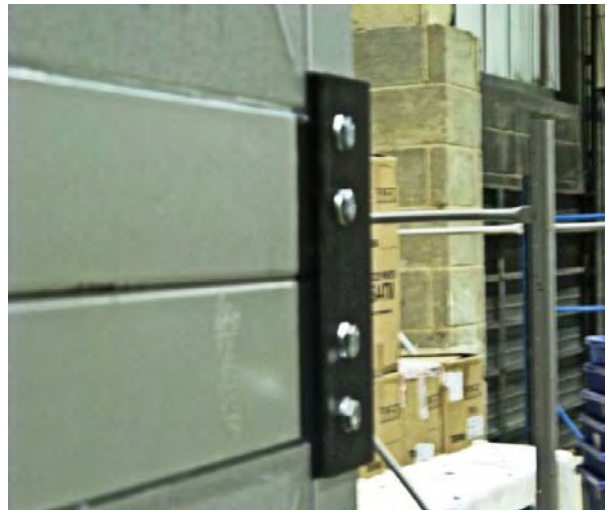
Once in place bolt together using angled brackets supplied.
