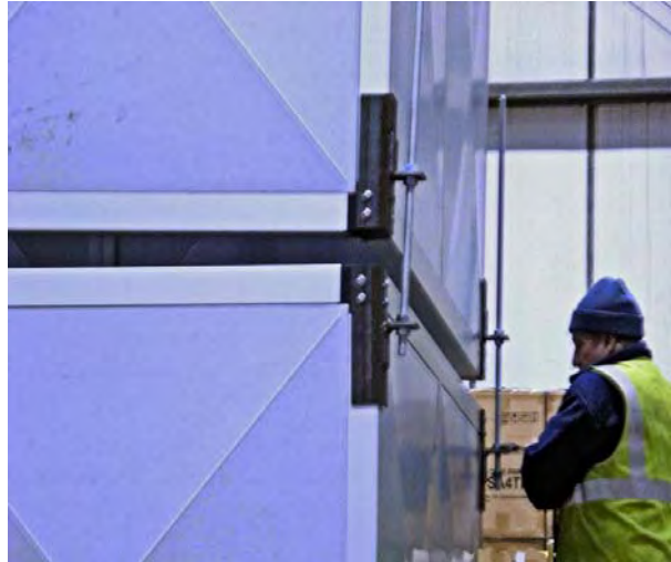
Lower top section corner by corner, keep space equal at all times.
