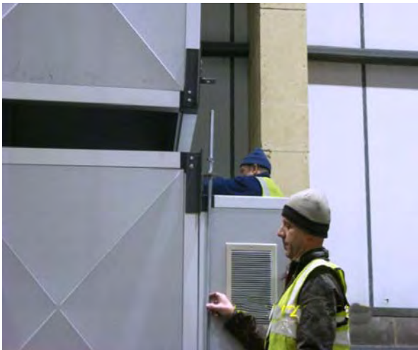
Use brackets and screwed rod supplied to support top section over lower section at each corner.
