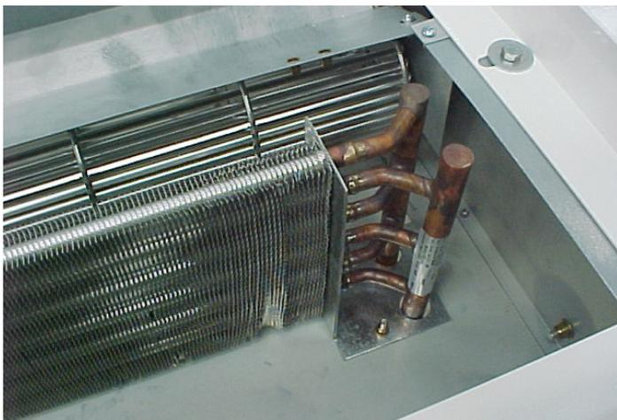
After fitting the coil and side supports fit the air deflector plate to the side supports and rotor cut-off plate using the screws provided.
