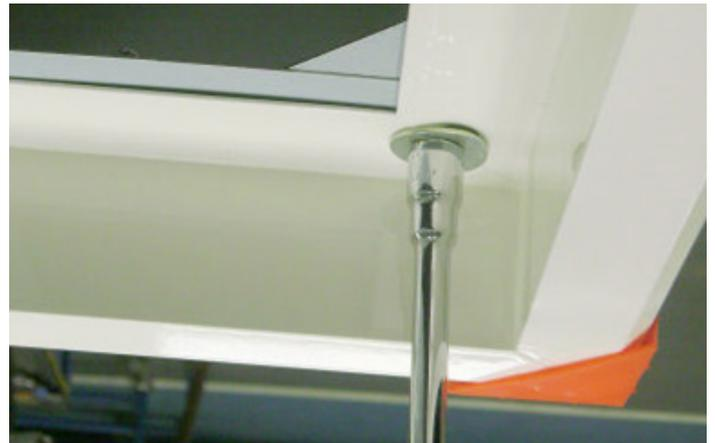
After fitting the product in the ceiling recess and adjusting the height to ensure that the grille sits flush to the ceiling (when re-fitted) take the grille assembly and refit using the screws removed during Step 5.
