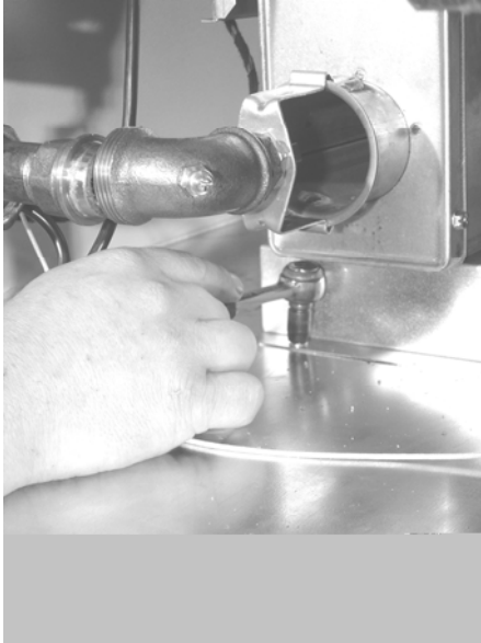
Figure 21 Remove 2 screws of the burner slider
