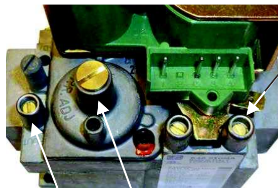
Injector pressure test point.
