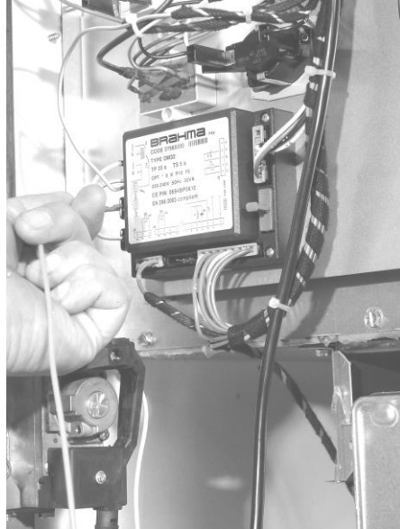
Figure 22 Disconnect wire of the ignition electrode at the burner controller
