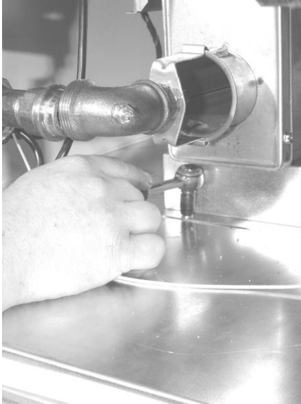
Figure 21 Remove 2 screws of the burner slider
