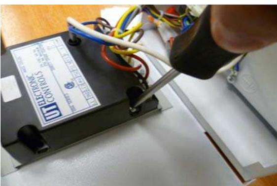
**Step 5:** Fit new burner controller
