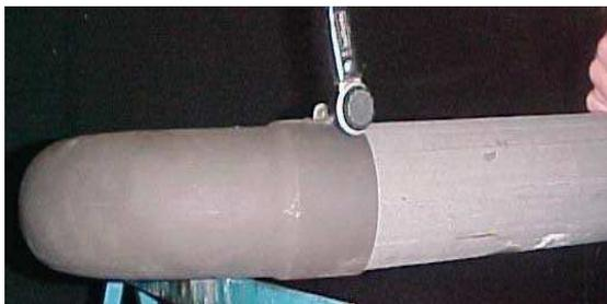
**Step 4:** Withdraw the turbulators from the appliance. Carefully note their condition and position. Replace turbulators if necessary.
