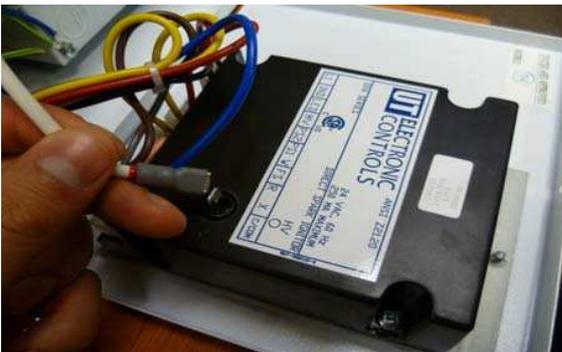
**Step 4:** Remove the two screws attaching the controller to the burner door and remove.
