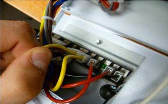
**Step 3:** Disconnect the HT Lead from burner controller.
